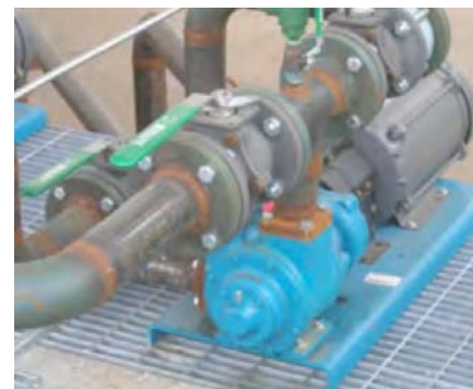
The pumps also have self-priming, high suction lift capabilities and explosion-proof motors.
